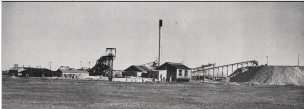
Figure 35 –The first mine shaft ever sunk along the Free State goldfields, namely the No. 3 Incline Shaft at the St. Helena Gold Mine (Felstar Publishers, 1968:151).
