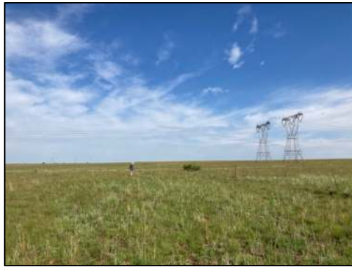
Figure 12 – View of existing powerlines.
