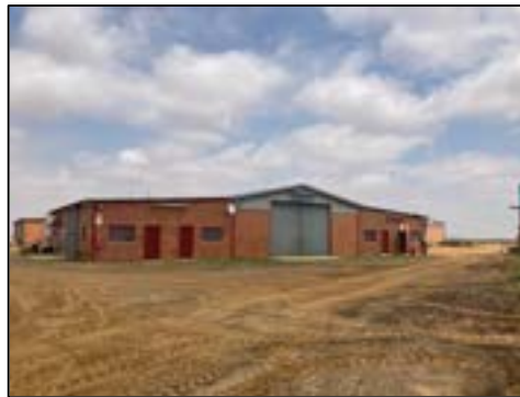
Figure 20 - New farm buildings close to proposed well location (west).
