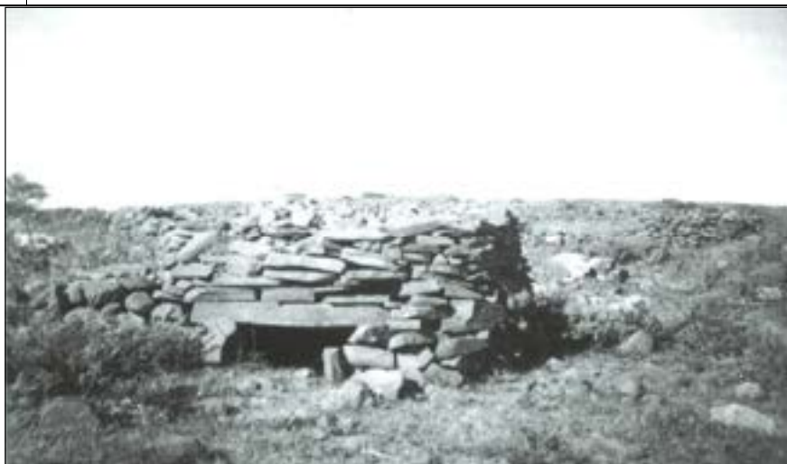
Figure 51 – Corbelled stone huts associated with a Type V settlement (Huffman, 2007:39).
