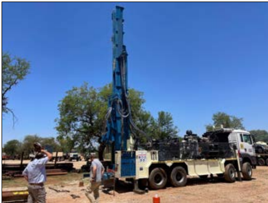
Figure 7 - Example of a drill rig (Source: Torque Africa).
