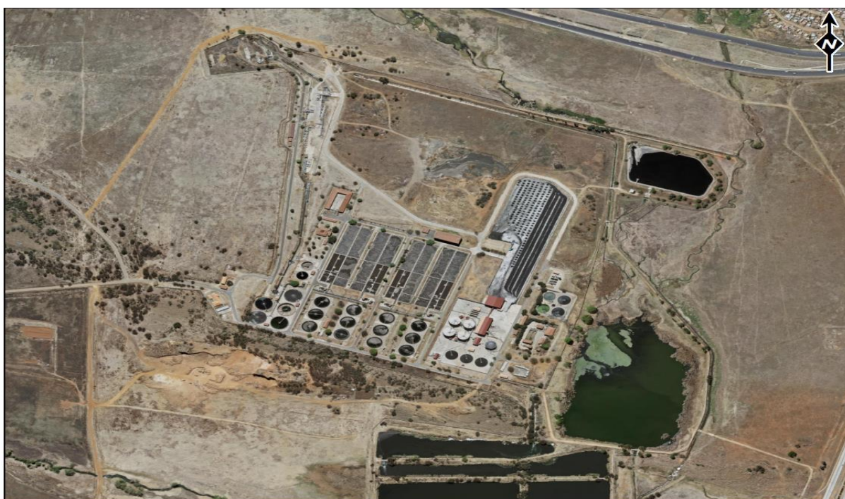
Figure 1-1: Location of the Bushkoppie WwTW
