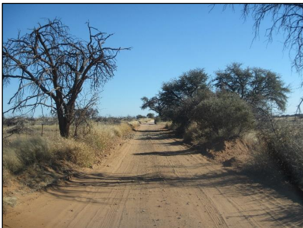
Figure 5: View along access road to be upgraded looking towards the northwest.
