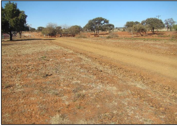
Figure 7: View along access road to be upgraded looking towards the southeast.
