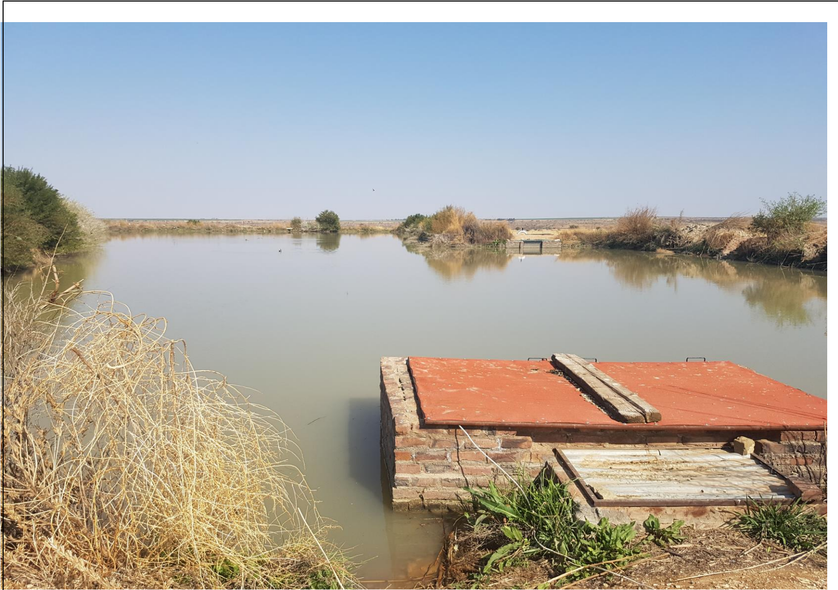
Figure 8: Existing Dam (29°34'45.27"S; 24° 5'18.61"E)
