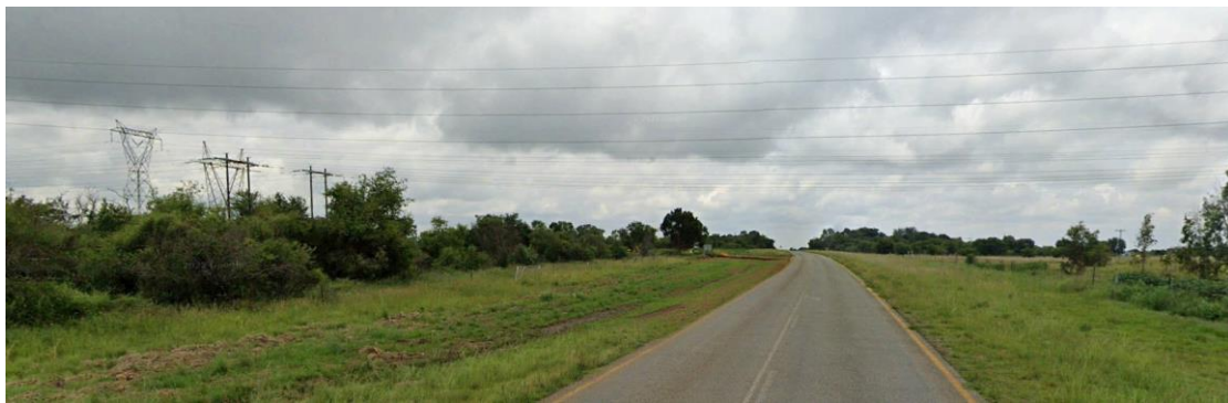
Figure 9: Power line infrastructure along the R505 arterial / main road.
