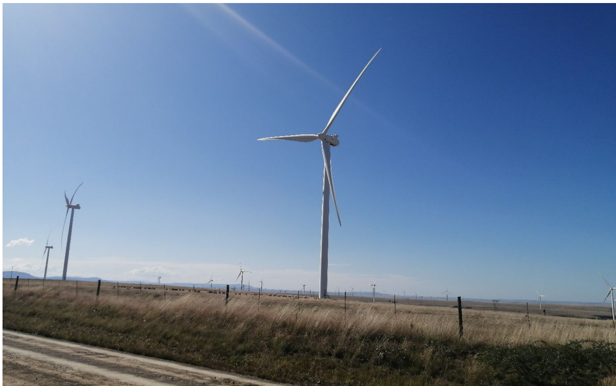
Figure 5: Site photography position 2 – Existing Wind Energy Facilities in the area
