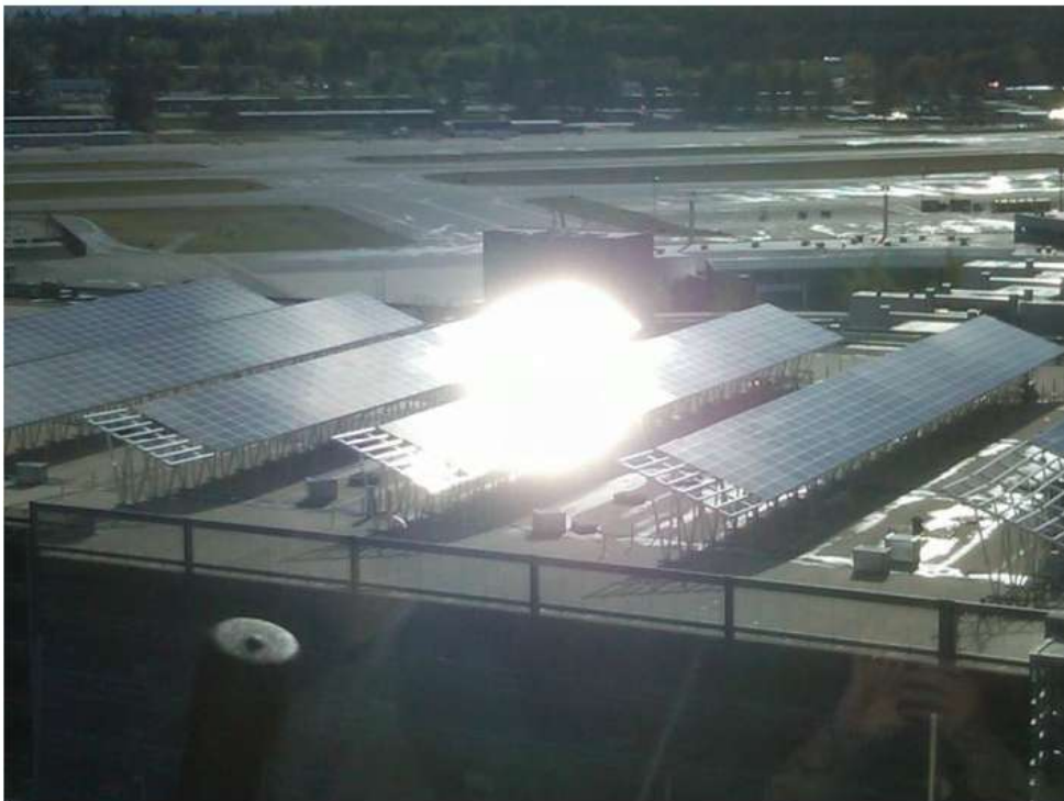
Plate 6, Glare experienced in the Control Tower at Boston Regional Airport from a PV array
