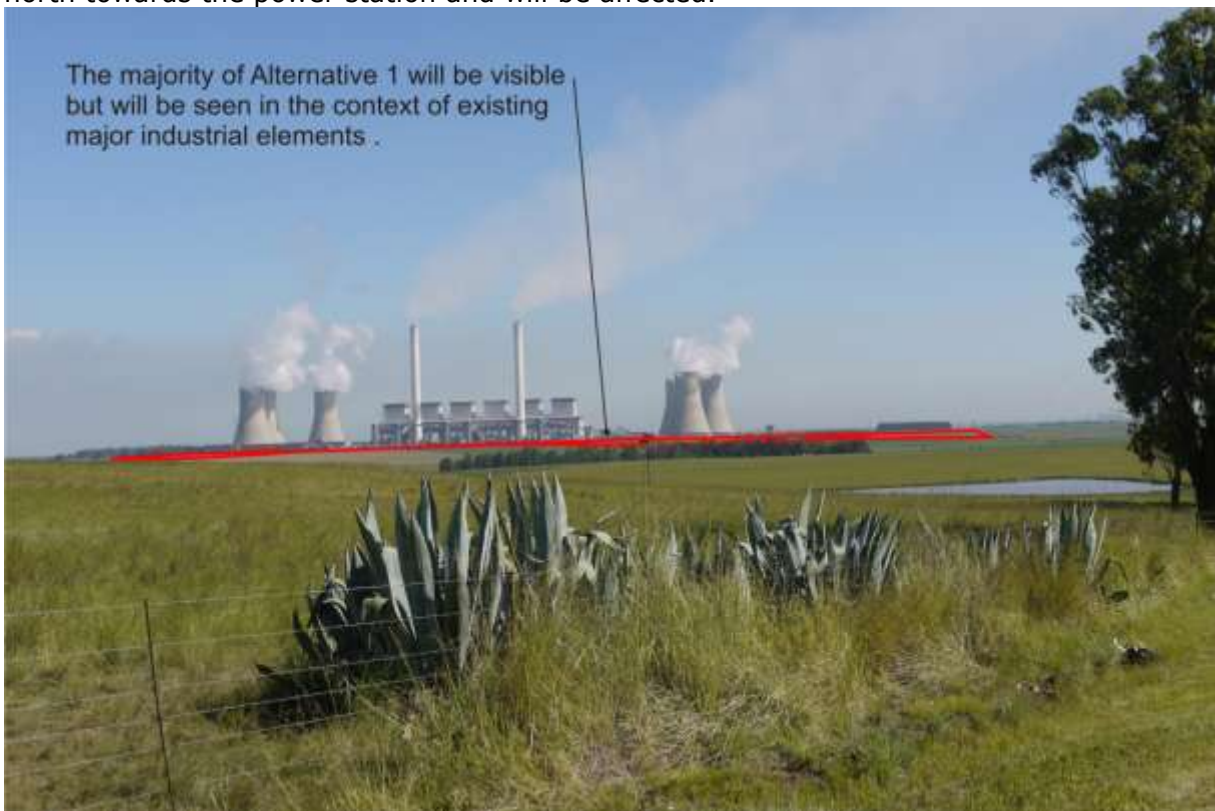
Plate 12, VP 5. View from the R38 and Farmstead to the south. Alternative 1 will be visible almost in its entirety but it will be viewed against the backdrop of the existing power station.
