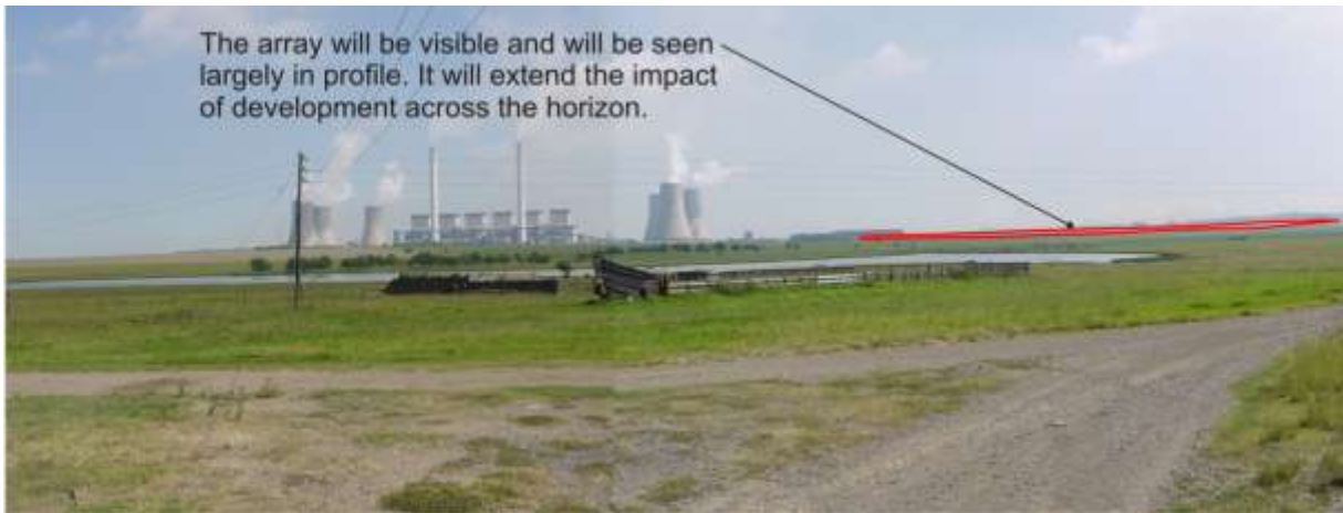
Plate 15, VP 6. View from a Farmstead to the south. Alternative 2 will be visible almost in its entirety. It will extend the extent industrial elements visible in the landscape.
