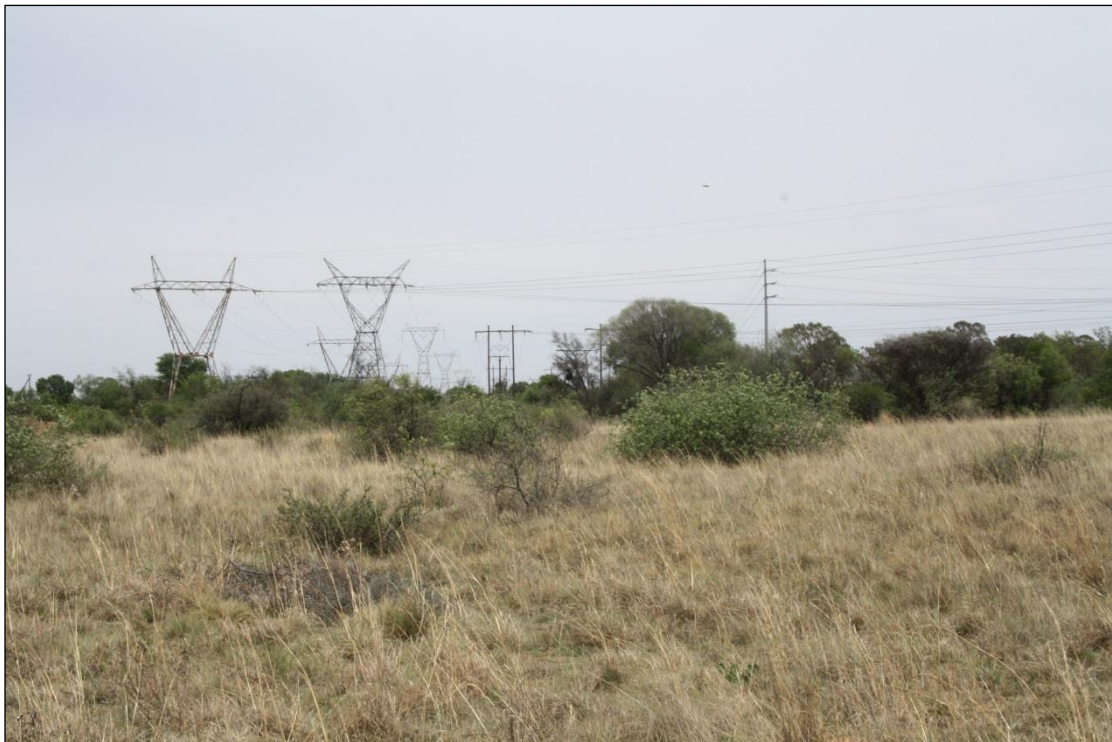
Figure 8: Power lines near the Watershed Substation.
