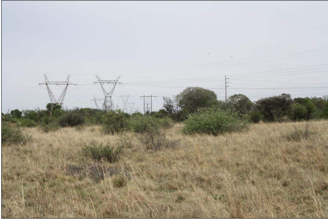
Figure 8: Power lines near the Watershed Substation.
