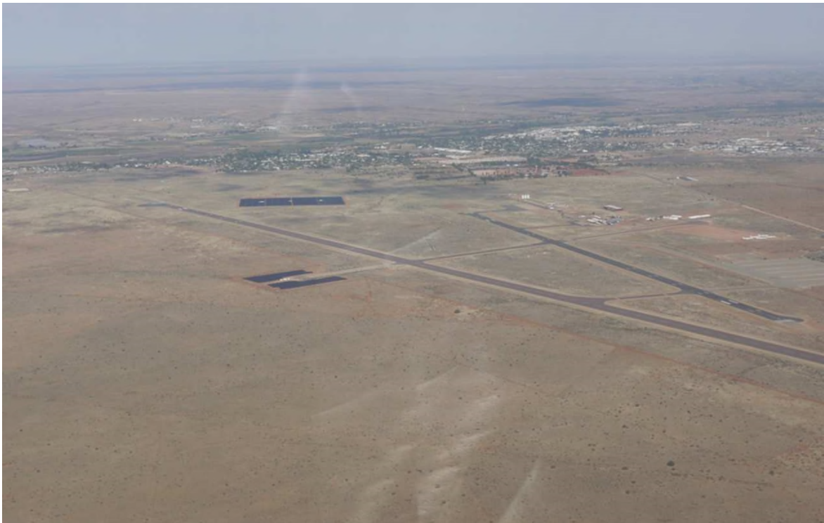
Plate 21 , Existing Solar Arrays at Upington Airport as seen from the air
