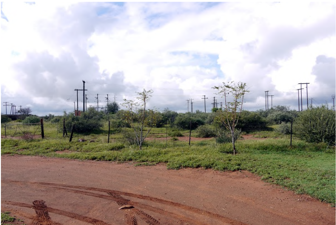
Plate 2, Existing Eskom MV overhead powerline on the northern boundary of the site. A number of alternatives are under consideration for the necessary grid connection which are subject to Eskom's plans for the construction of a new substation (Bophirima) in the area indicated as well as a new 132kV overhead power line link to the existing Mookodi Substation.
