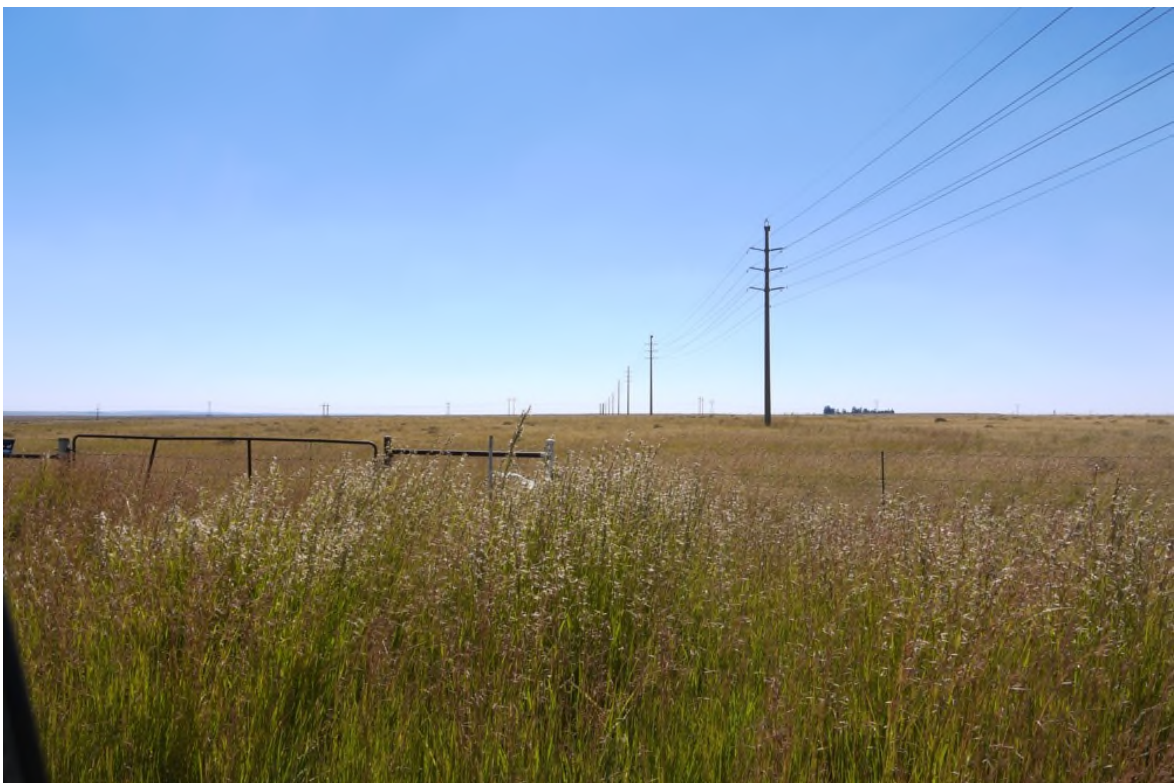
Plate 25, View of a 132kV overhead power line similar line to that proposed. Note pylons on the horizon (approx 2.5km distance) are just visible.
