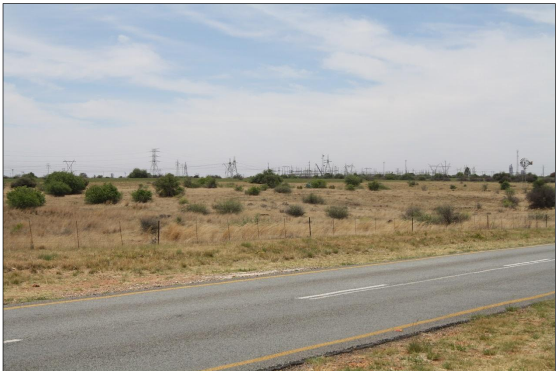
Figure 7: The Watershed Substation viewed from the R505 Arterial Road.
