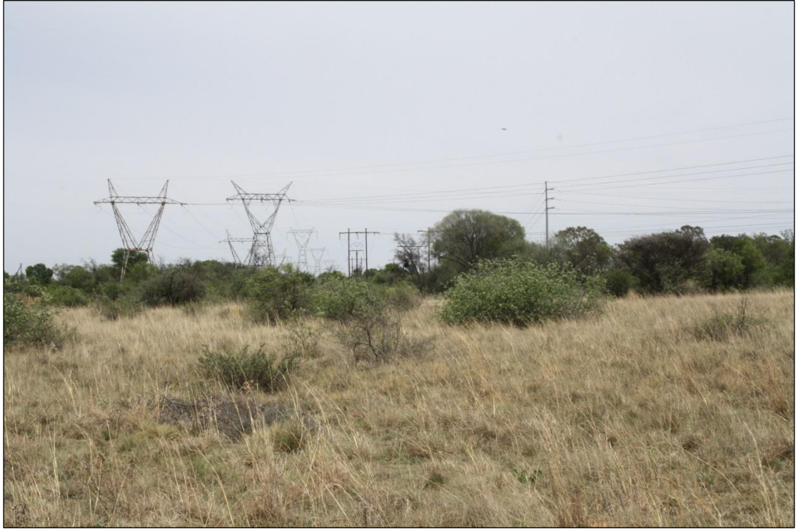
Figure 8: Power lines near the Watershed Substation.
