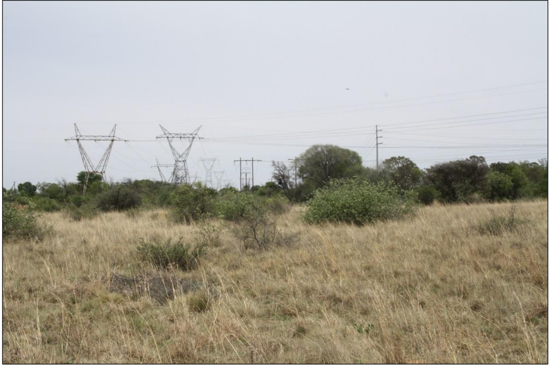
Figure 8: Power lines near the Watershed Substation.
