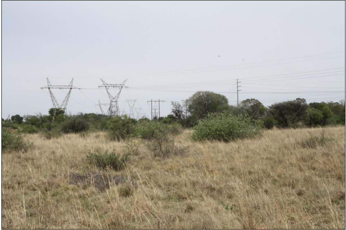
Figure 8: Power lines near the Watershed Substation.
