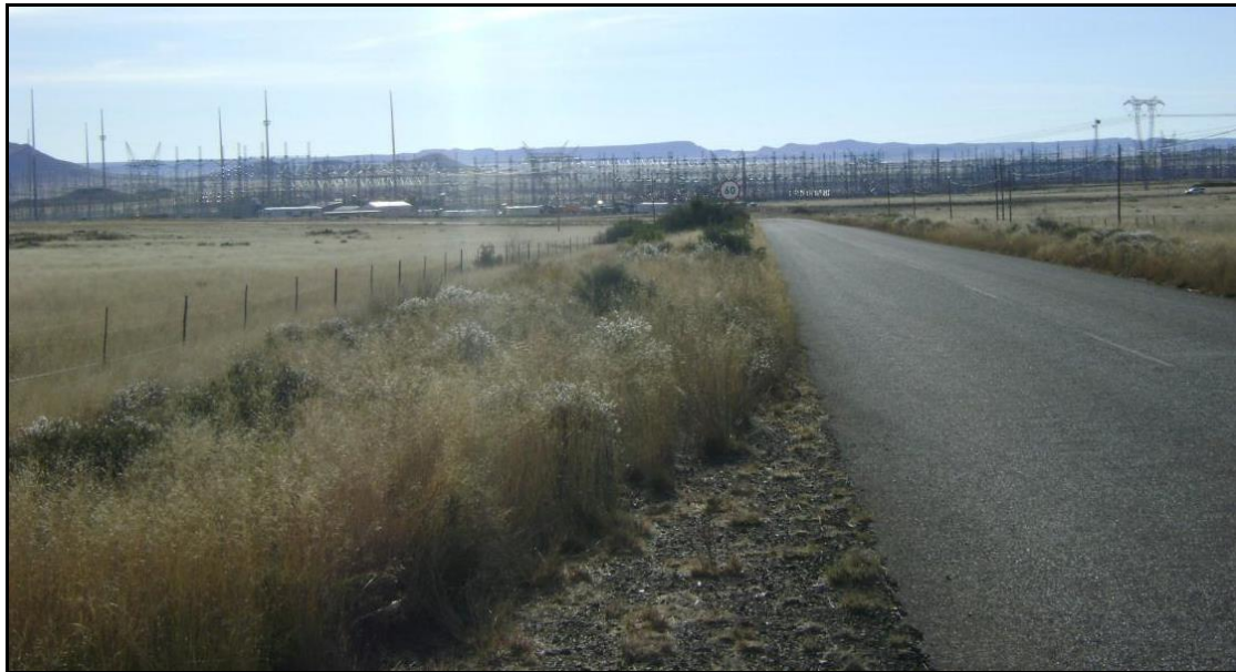
Figure 8: The Hydra Substation in the west of the study area.
