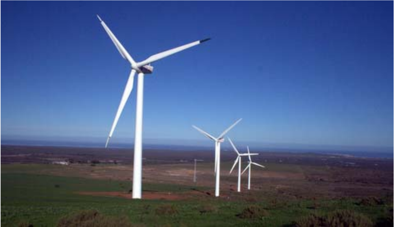
Figure 3: The Darling Wind Energy Facility in the Western Cape Province, South Africa
