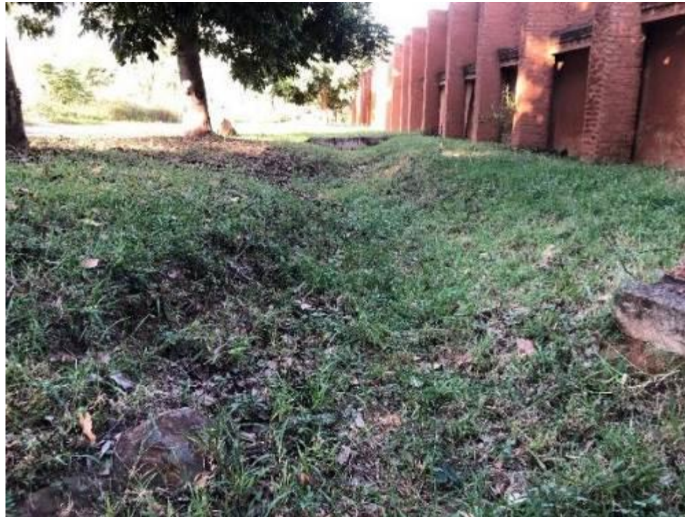
Figure 18: The Drainage Line on Erf 349.
