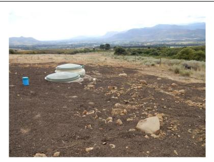
Figure 7.3 Above ground component of the BioDisc domestic sewage treatment plant (BA model), located at the Tented Camp site.
