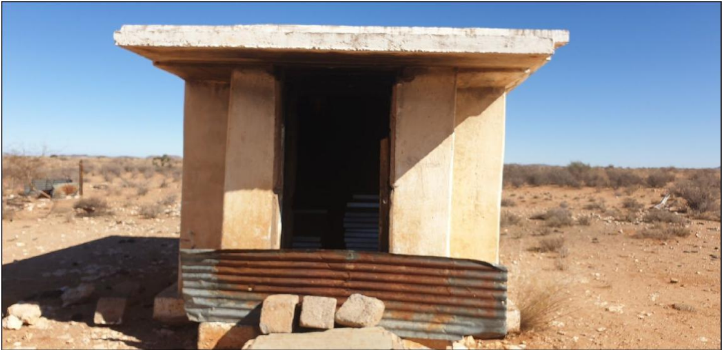
Figures 6.16 Store room or machine room associated with the historic tungsten mine (Pt 21)
