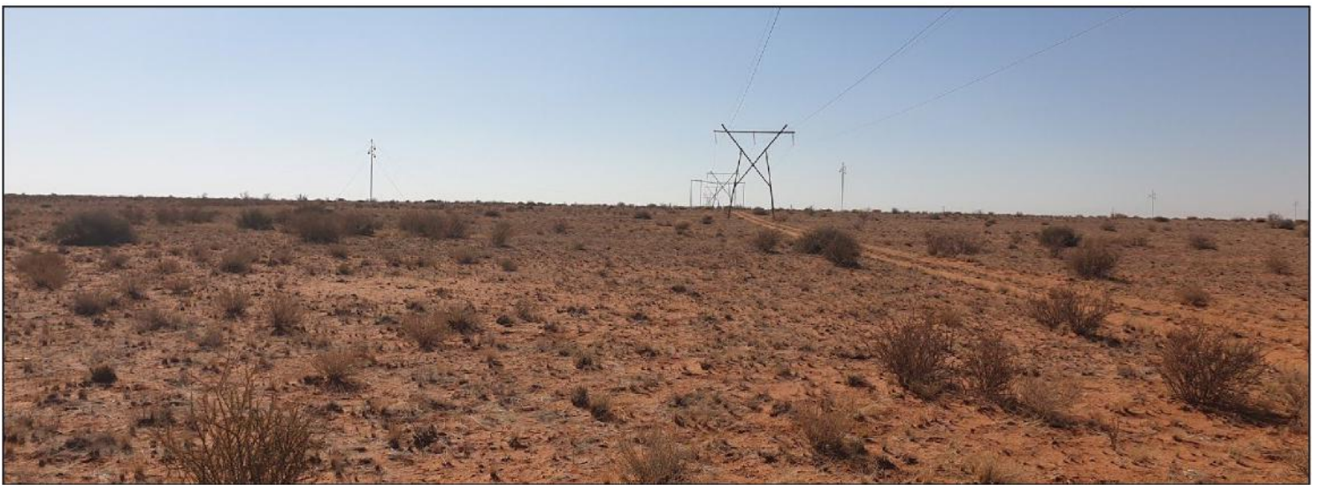
Figure 4.11: Contextual Images of existing OHL's View from east towards the west
