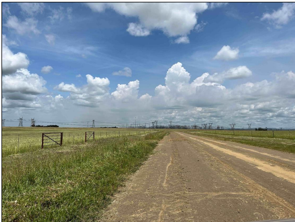
Figure 17: Zeus Substation south-west of the Mukondeleli WEF project area.
