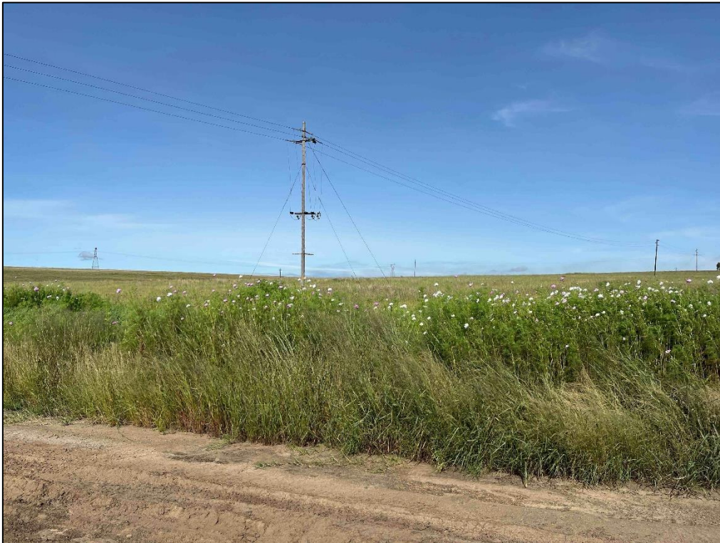
Figure 22: View west from Viewpoint MW2 - Pre-Construction
