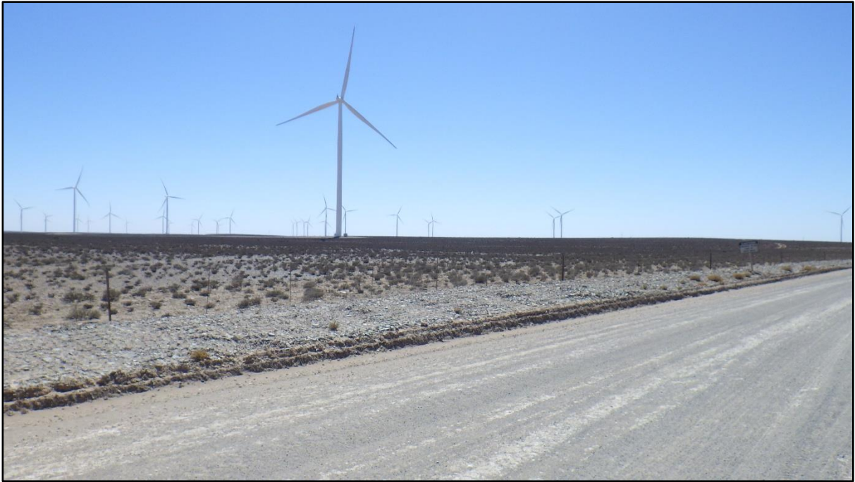
Figure 2: Wind turbines at Loeriesfontein 2 WEF in the Northern Cape Province.
