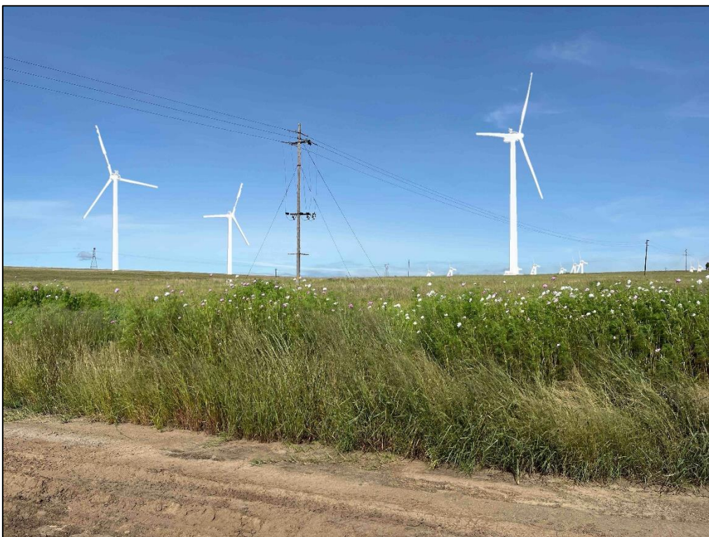
Figure 23: View west from Viewpoint MW2 - Post-Construction
