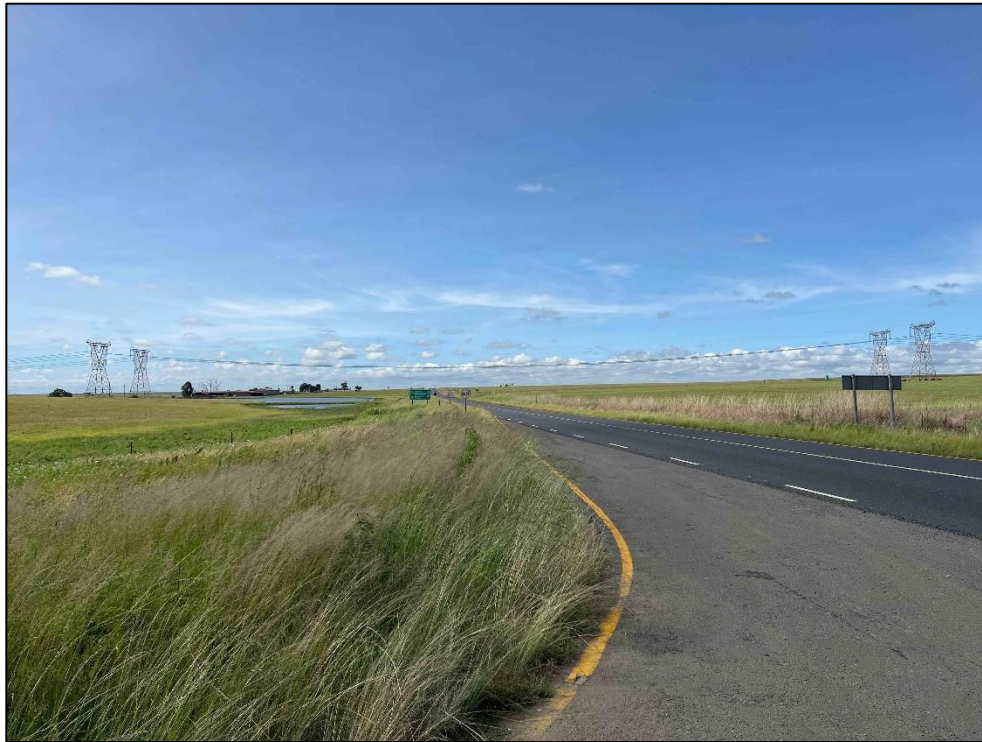
Figure 18: 400kV power lines High voltage power lines to the south of the Mukondeleli WEF project area.
