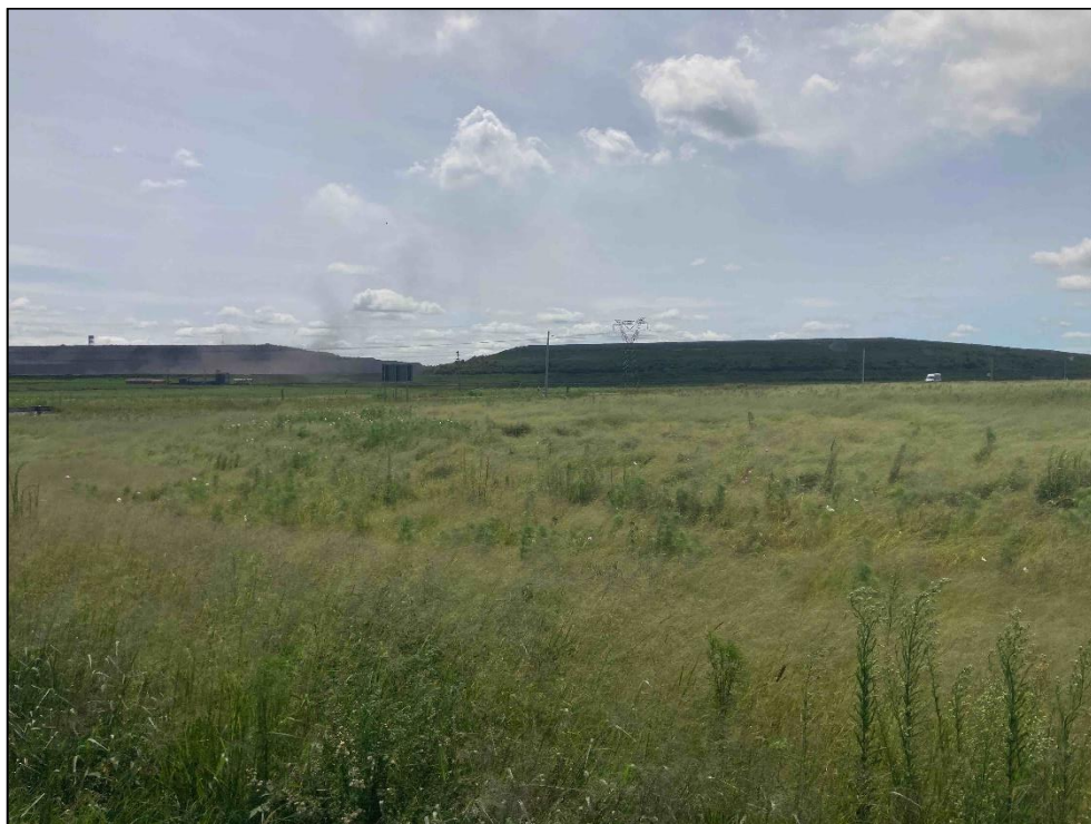
Figure 13: Coal dumps adjacent to the Sasol Fuel Plant
