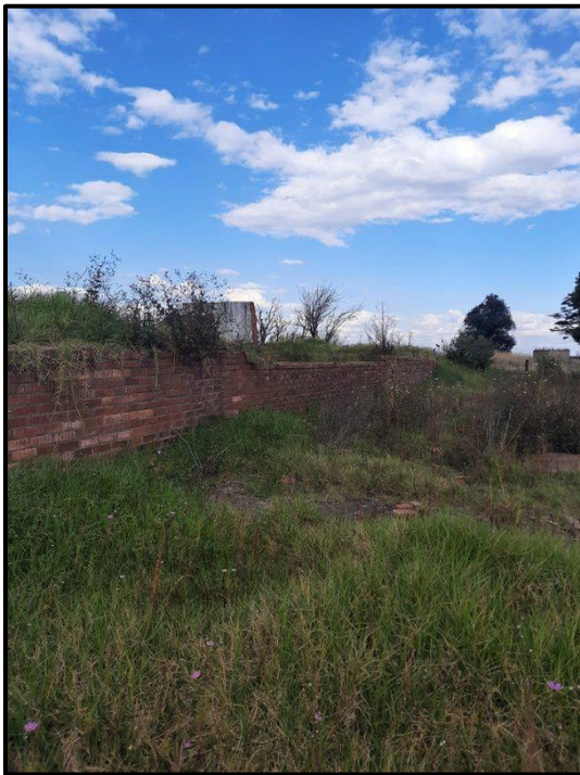
Figure 8.8. Brick structures at Waypoint 097.
