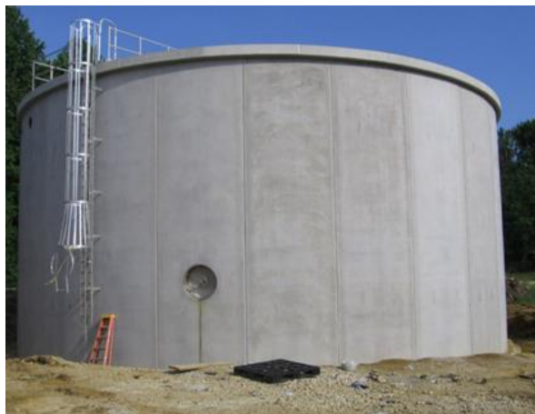
Figure 4-3: Typical water reservoir (left concrete, right steel tank ~ 6m).
