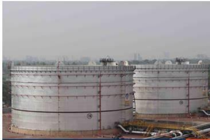
Figure 4-9: Double-deck floating roof storage tank
