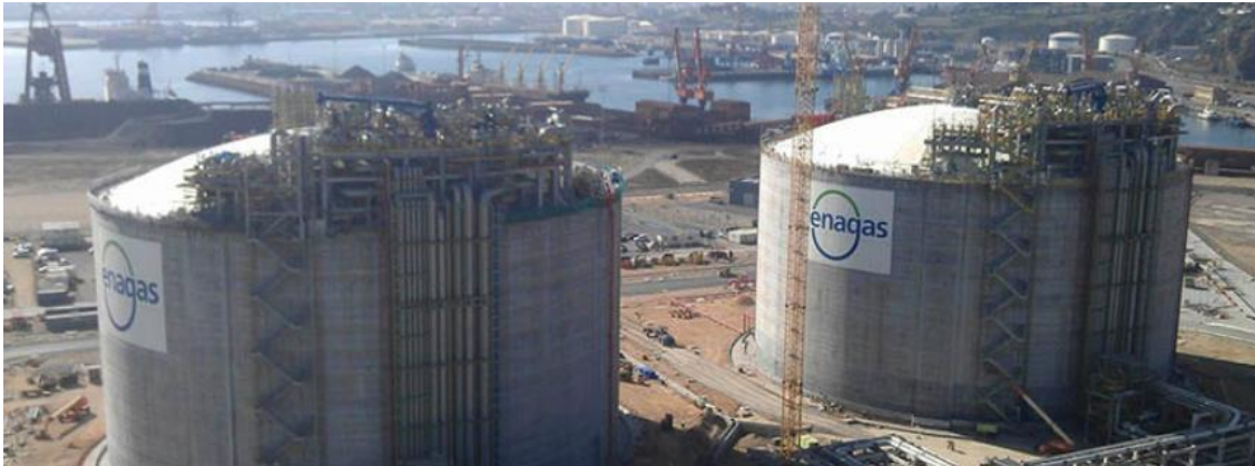
Figure 4-12: Liquid Ammonia Storage system (Energas example).
