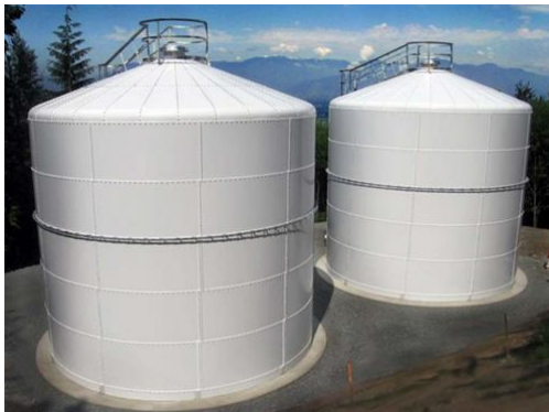
Figure 4-8: Single-walled fixed storage tanks (left and double-walled fixed roof tank (right)
