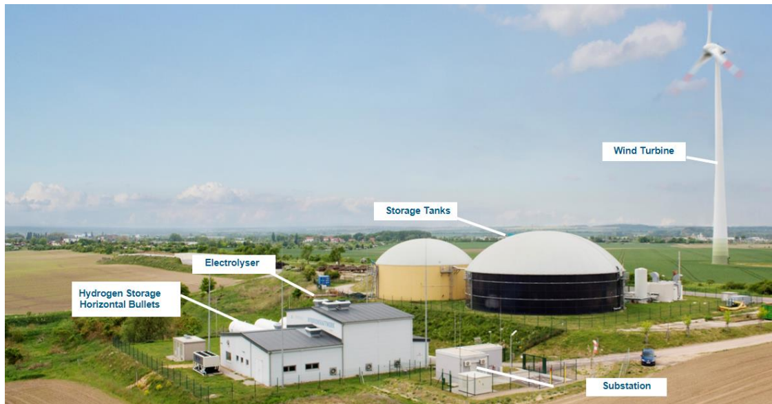
Figure 4-2: Closer View of Electrolyser Housing and Storage Tanks
