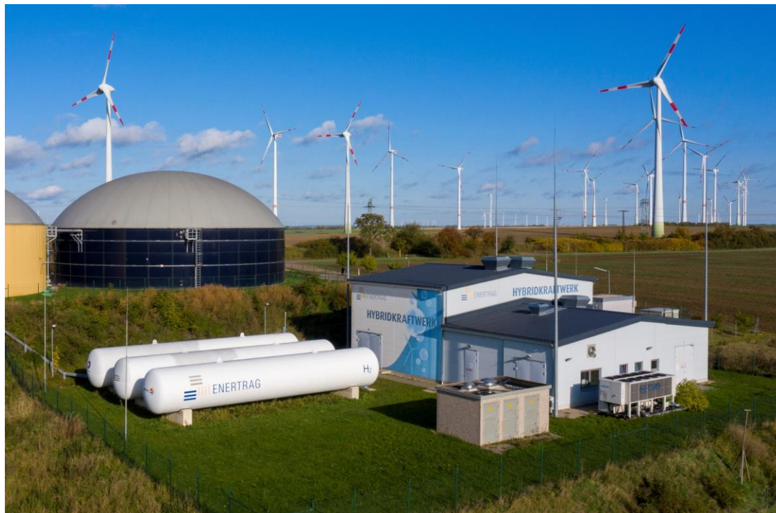
Figure 4-2: Closer View of Electrolyser Housing and Storage Tanks
