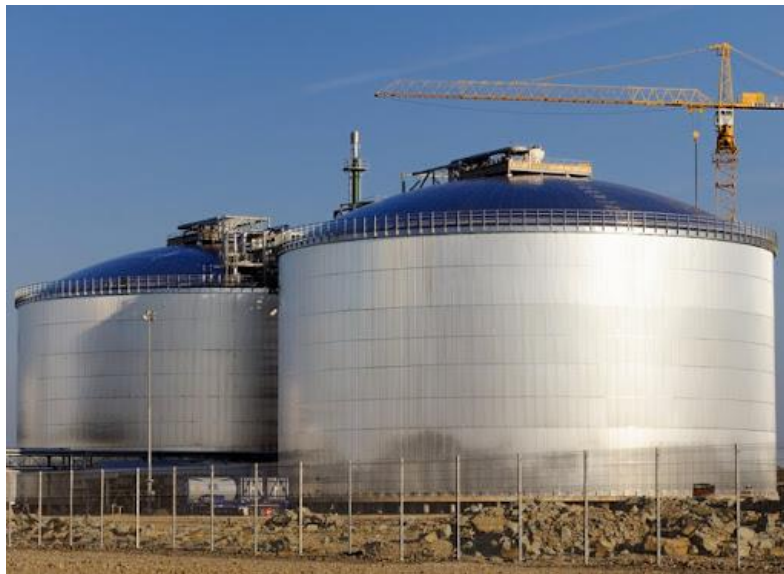
Figure 4-13: Cryogenic ammonia storage tanks
