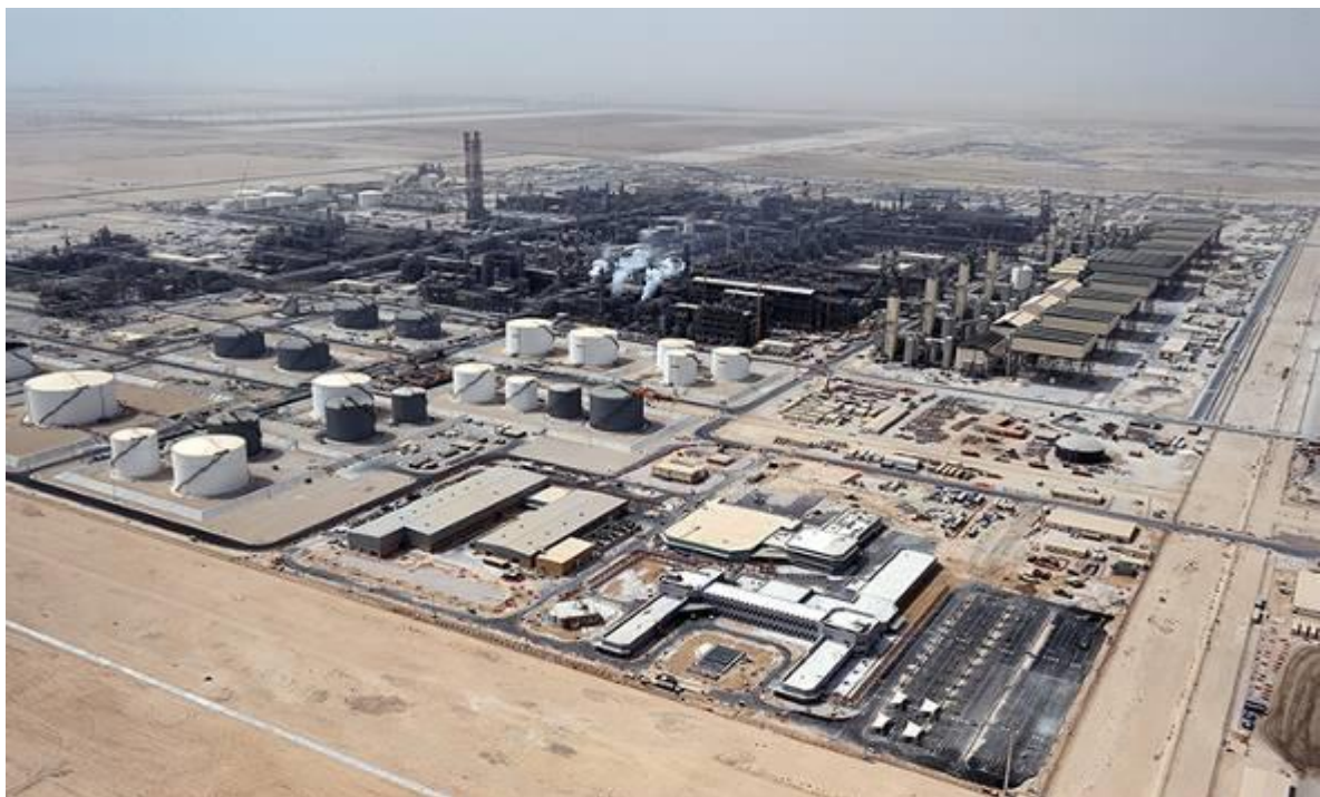
Photograph 3.1: Secunda Sasol Facility
