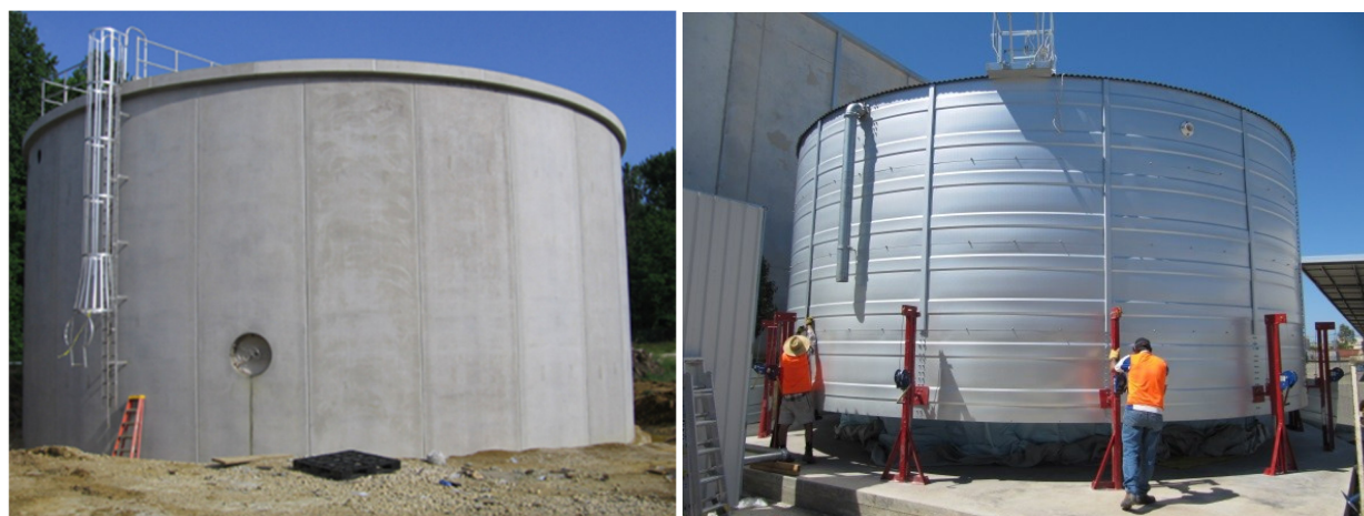
Figure 3-1: Typical water reservoir (left concrete, right steel tank ~ 6m).
