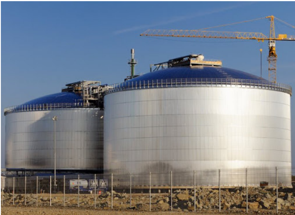
Figure 3-6: Cryogenic ammonia storage tanks
