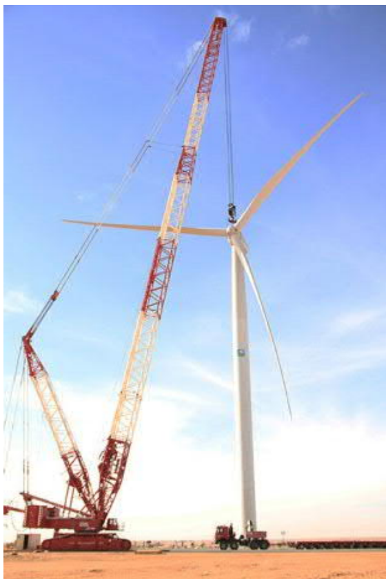
Figure 4-7: Crawler Crane used to assemble turbine (Liebherr, 2017)
