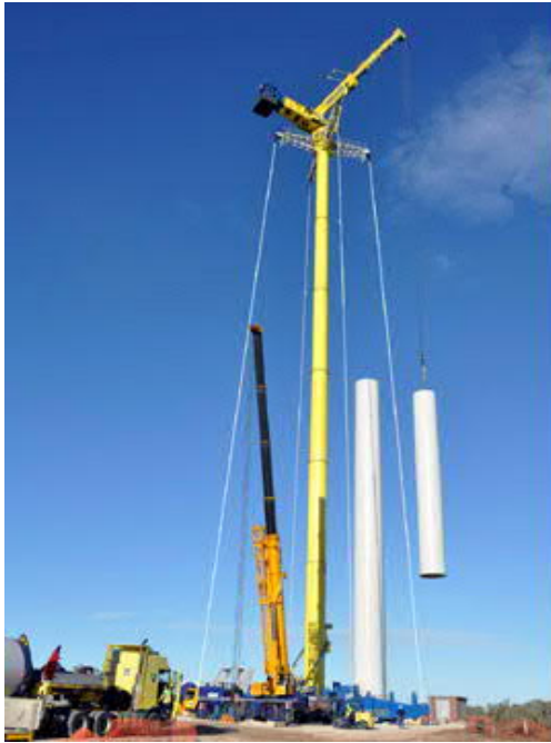
Figure 4-8: Cranes at work
