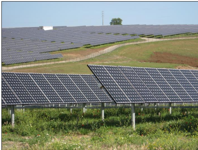
Figure 1.2. Photovoltaic (PV) energy facility.
