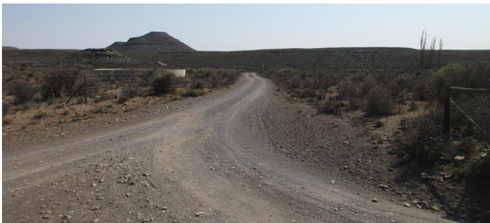
Figure 19 - Access to Mura SEF 1 & 2
