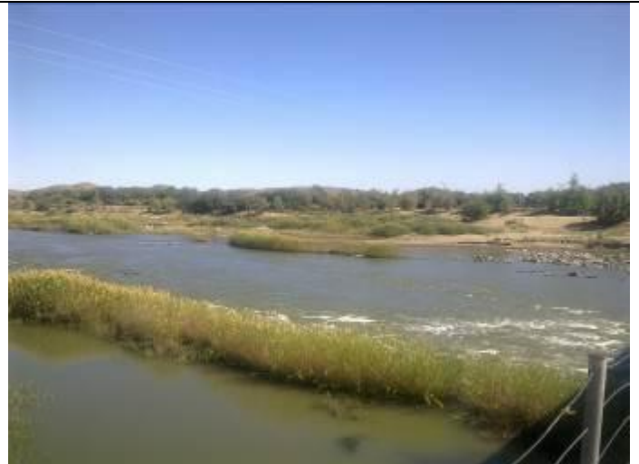
Figure 15: Downstream view of the C3 site showing the rocky rapids downstream of the crossing.
