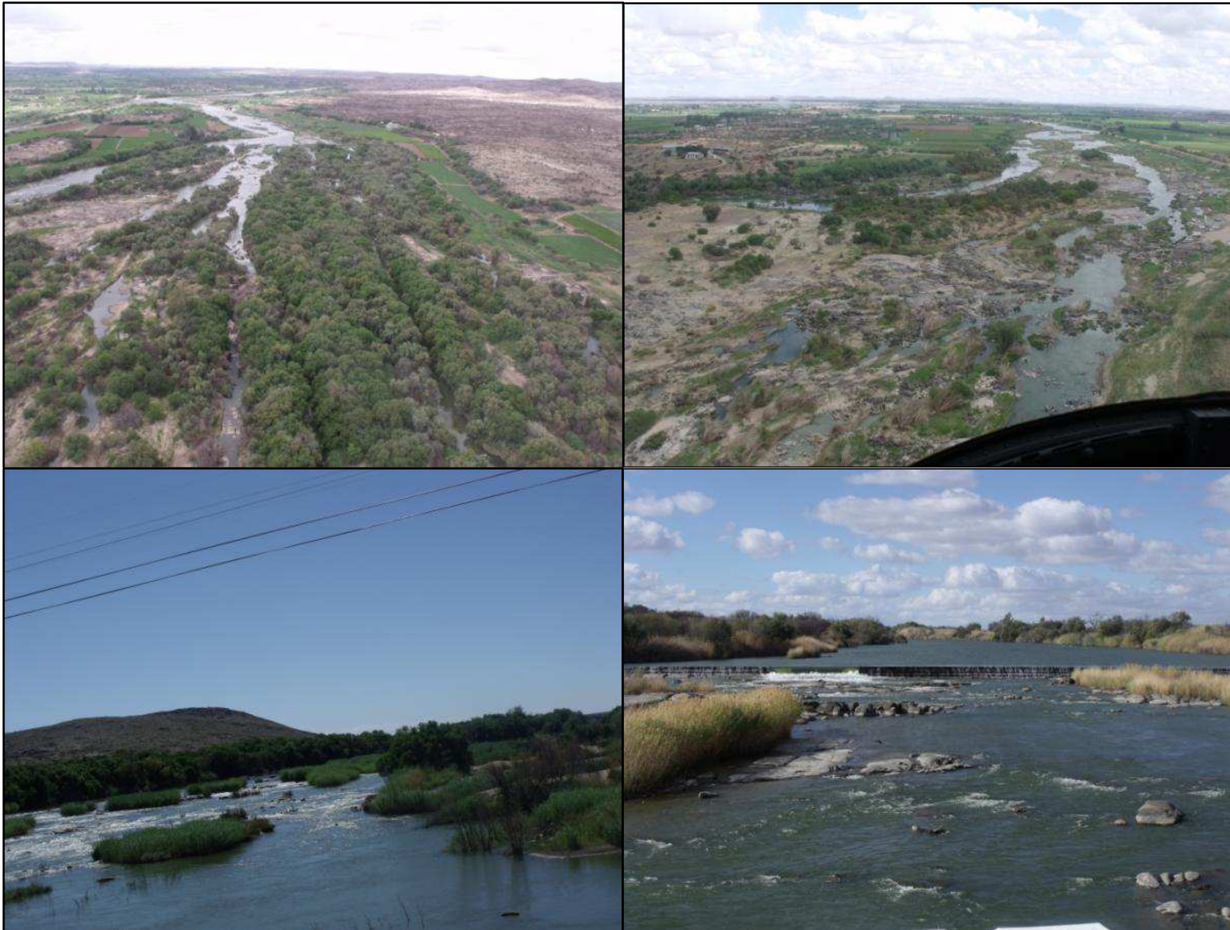
Figure 5-4: Proposed River Crossings not recommended (Aries 2 (top left), Nieuwehoop 3 (top right), Aries 3 (bottom left) and Nieuwehoop 2 (bottom right))
