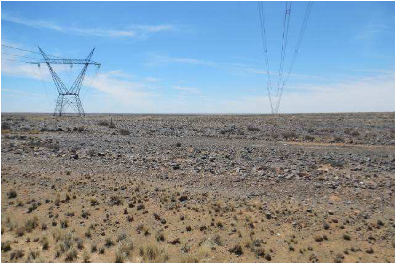
Figure 17: Existing transmission lines at Aries substation.
