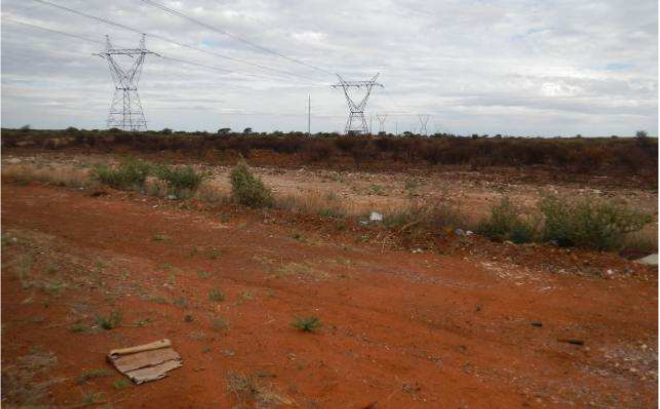
Figure 9: Existing transmission lines near Kathu.
