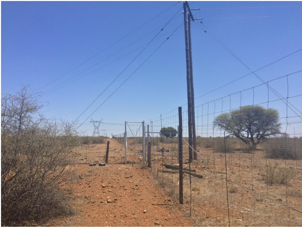
Figure 8: View towards Vryburg and Eskom infrastructure
