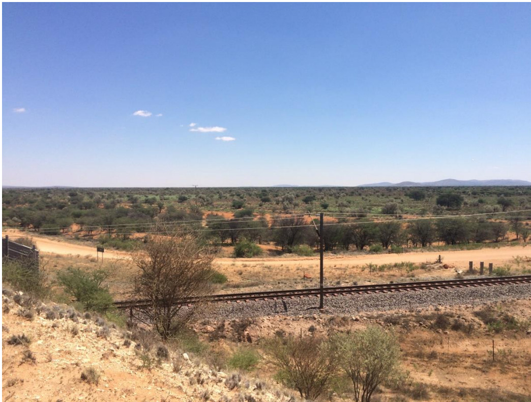
Figure 8: View of area from bridge towards a northern direction
