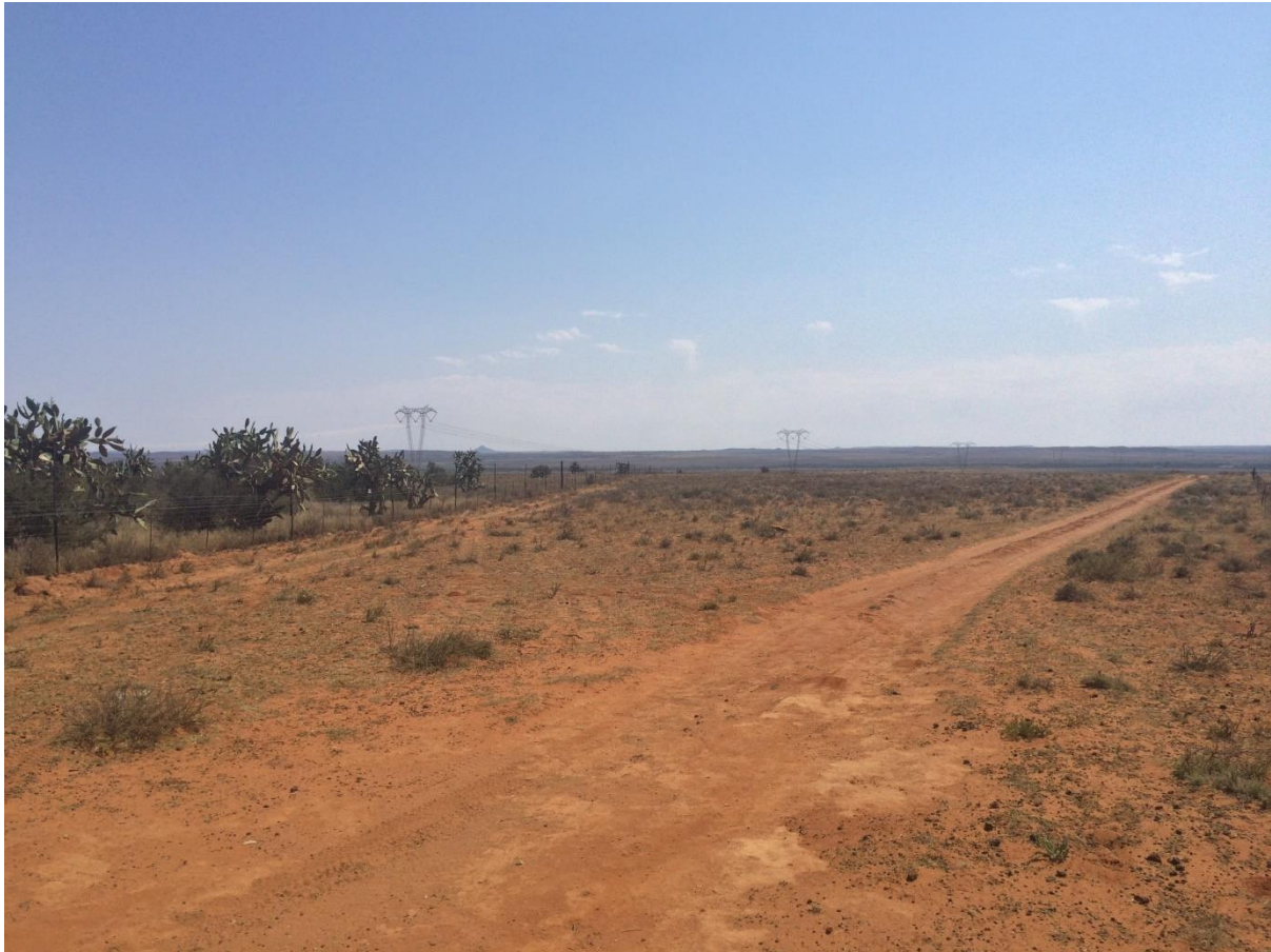
Figure 3: View of existing Eskom power line infrastructure
