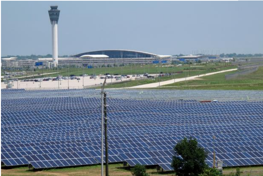
Figure 12: The Indiana Solar Farm at the Indianapolis International Airport
