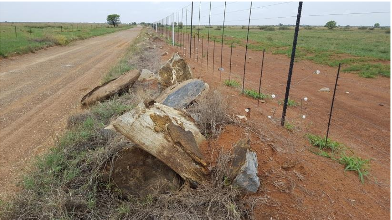
Figure 5. View near the site of hard, shallow underlying dolomite rock that has been excavated during the planting of fence poles. Such rock appears to underlie the whole site at a depth of between 40 and 120cm.
