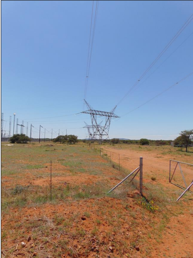
Photograph 1.4.4. Overview of the Eskom transmission lines running along the proposed sites.
