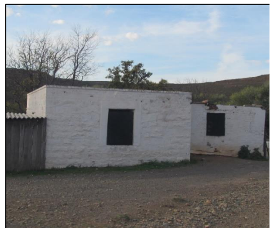
Figure 44: Structure in the Leeukloof Farm complex at Waypoint 1850. Source: Orton (2021a: fig. 50).
