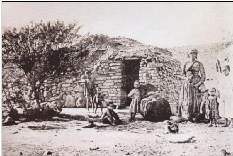
Figure 21: A shepherd's hut photographed near Beaufort West in the early 20th century. Note the low, narrow doorway and informal roof structure. Source: Schoeman (2013:48).
