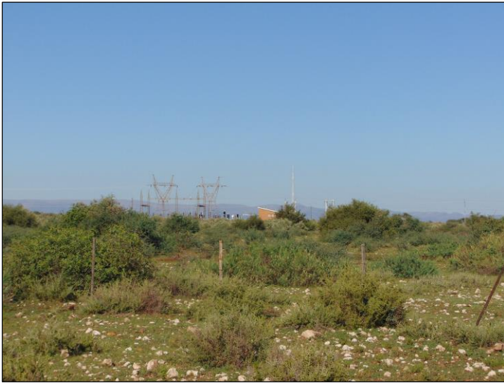
Photograph 1.4.6. Eskom substation South West of the Boitshoko SPP site.
