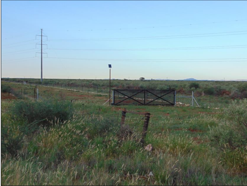
Photograph 1.4.1. Overview of the proposed Boitshoko SPP from the main road (R380) in a Southern direction.
