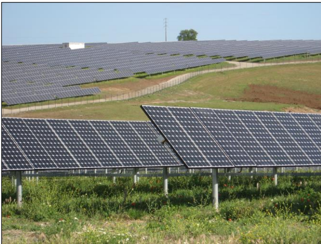
Figure 1.2. Photovoltaic (PV) energy facility.
