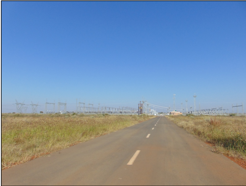
Photograph 1.4.4. Overview of Eskoms' Mookodi Substation located next to the N18 national road, about 5km South of Vryburg.
