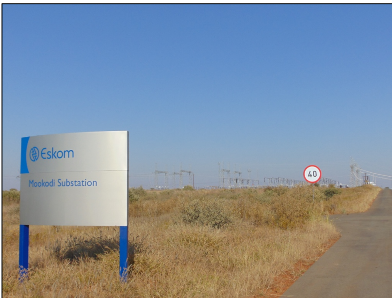
Photograph 1.4.3. Overview of Eskoms' Mookodi Substation located next to the N18 national road, about 5km South of Vryburg.
