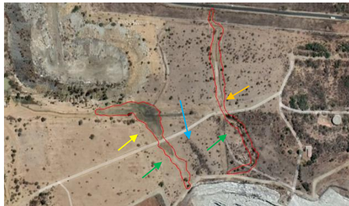
Figure A: The informal gravel road (blue arrow) has led to ponding upgradient of the road (green arrows) and desiccation and channel straightening downgradient thereof (orange arrow). Ponding (yellow) in the UCVB wetland is also caused by the WRD.
