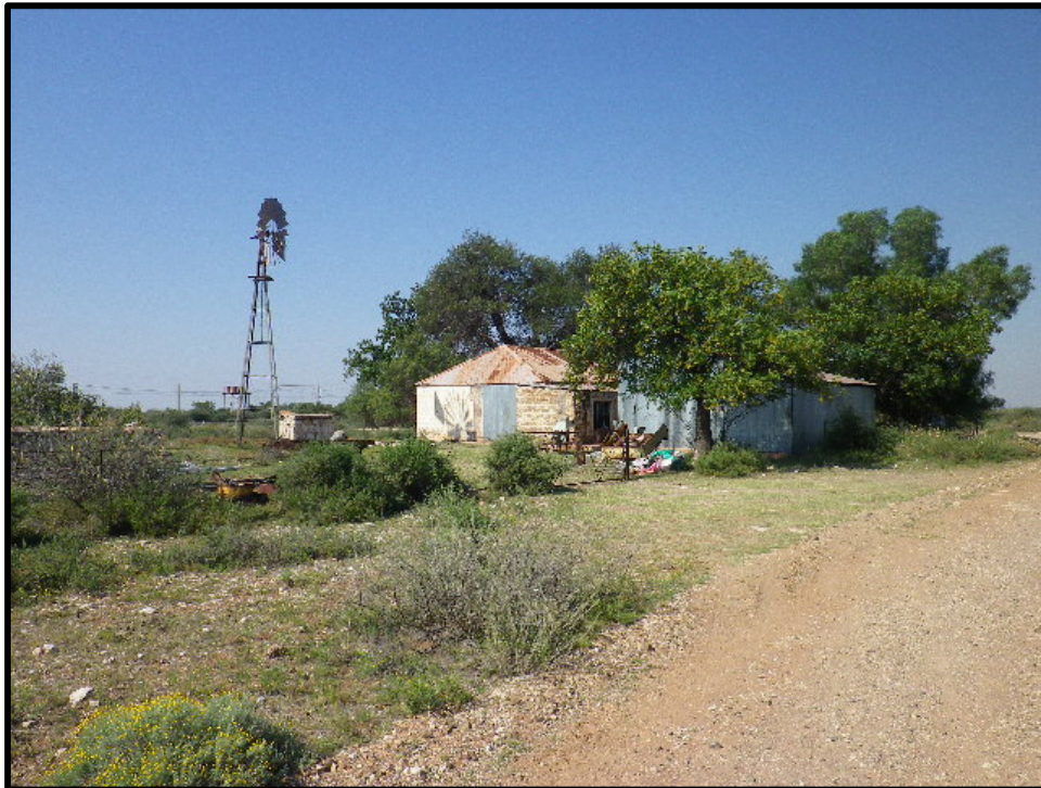
Photograph 3.3: Old farm buildings on the site
