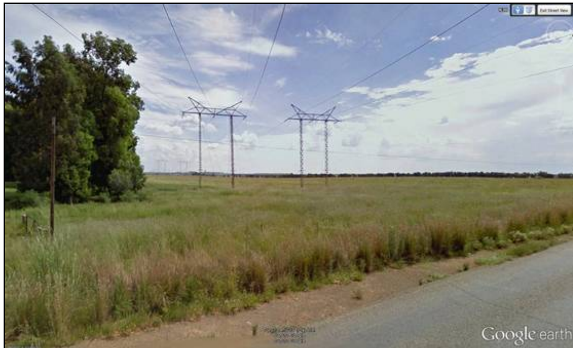
Figure 2: Google Earth Street View of the proposed development site from the R30 (with the Theseus-Oryx 1 and Beatrix-Theseus power lines in the foreground).
