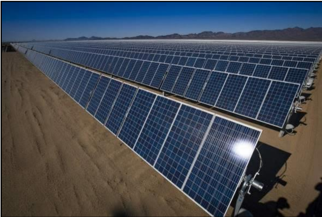
Photograph 1.1: Typical PV SEF facility
