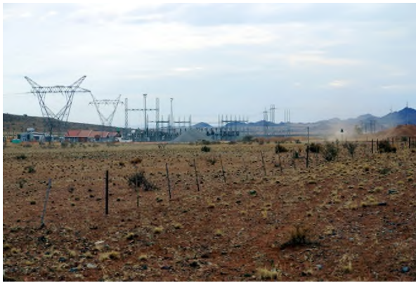
Plate 5, Industrial Landscape Character Area. Paulputs Substation.
