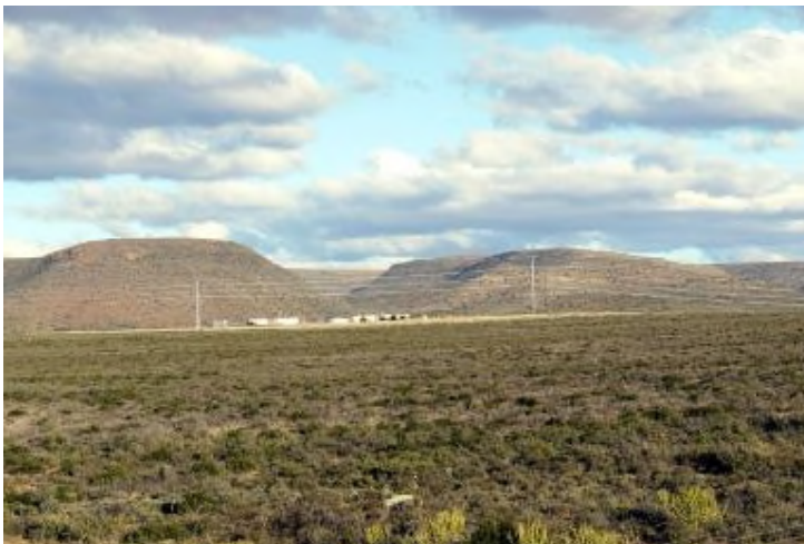
Plate 2, Eskom 220kV Monopole.
