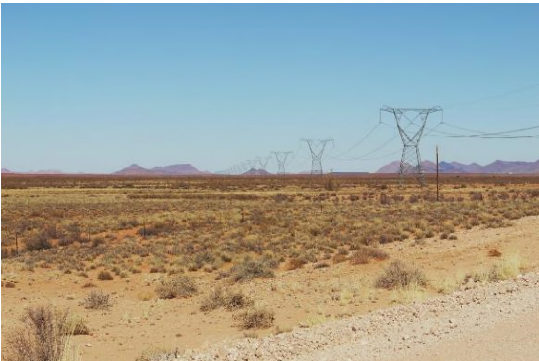
Plate 18, VP 2 – View looking to the west along the existing 400kV Aries-Aggenais
