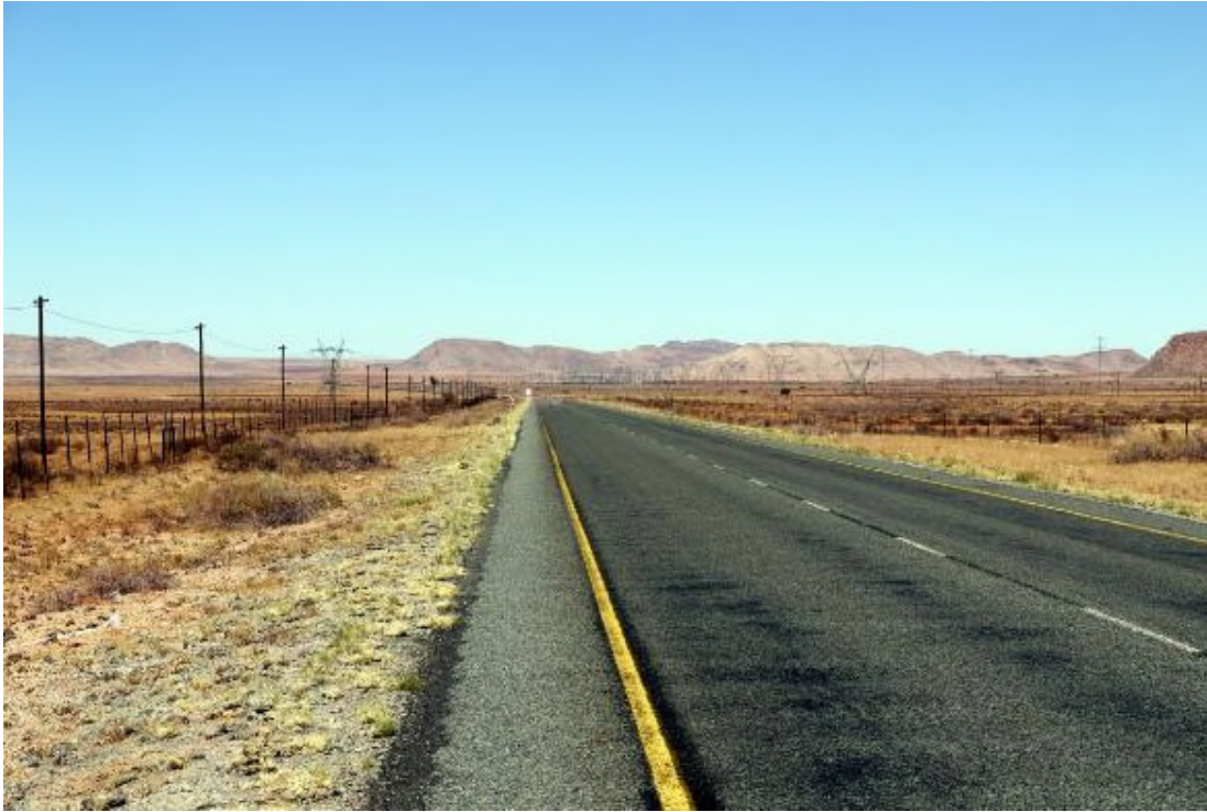
Plate 22, VP 6 – View looking to the south west along the N14 from close to Aggeneys. At this position major existing electrical infrastructure is obvious on both sides of the road. The proposed Geelstert Grid Connection Corridor Line Corridor will be centred on the N14 at this location.
