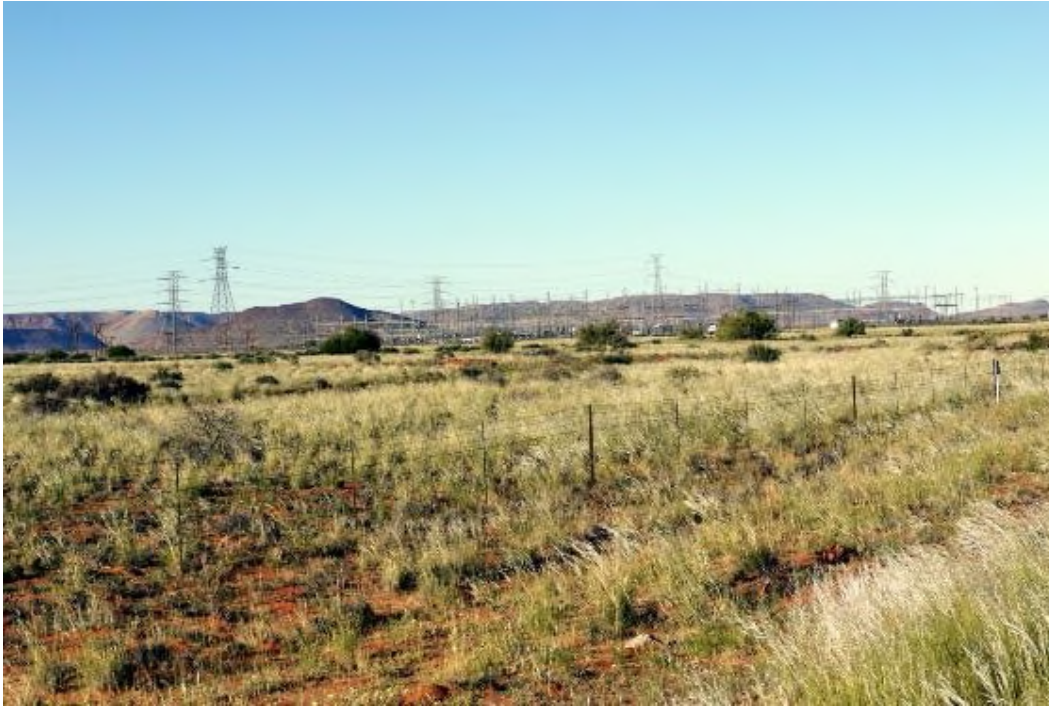
Plate 1, Existing Aggeneis 400/132kV Main Transformer Substation (MTS).
