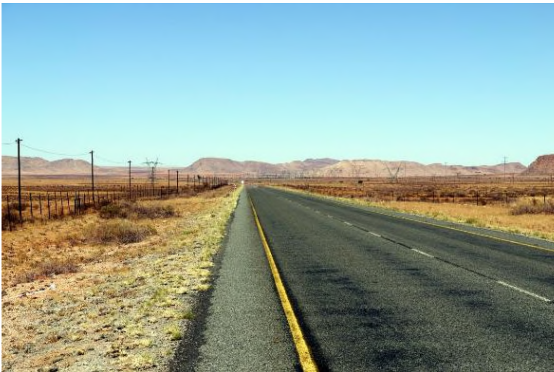
Plate 7, Views of the Aggeneis to Aries 400kV power line crossing the N14 to the south of Aggeneis. The view is looking towards the Aggeneis MTS from close to the point where grid connection corridor runs parallel to the N14.
