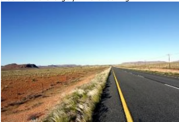
Plate 13, The N14. This is a major regional route that runs to the west of the proposed project area. It is an important regional tourism route
