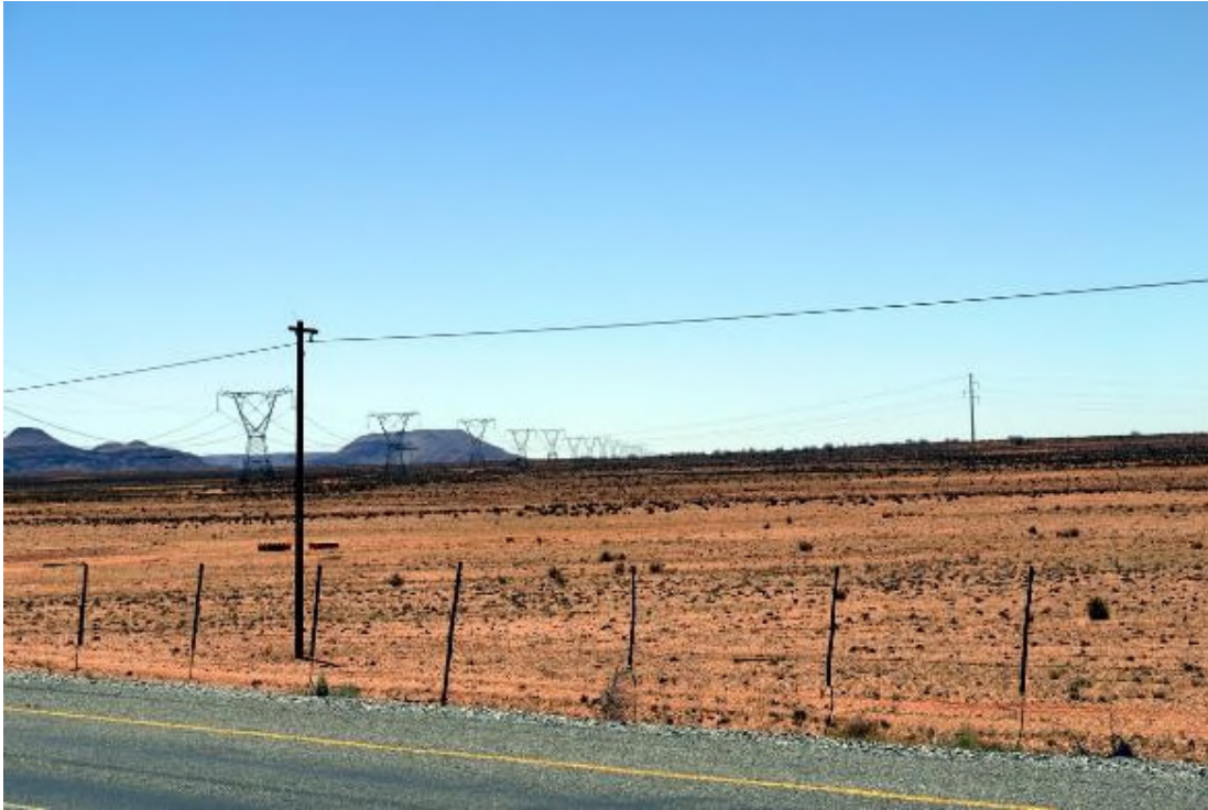
Plate 8, Views of the Aggeneis to Aries 400kV power line and the Geelstert Grid Connection corridor approaching the N14 from the direction of the proposed Geelstert 1 and Geelstert 2 solar PV facilities. The proposed grid connection corridor for the Geelstert Grid Connection is located to the right of this existing power line.
