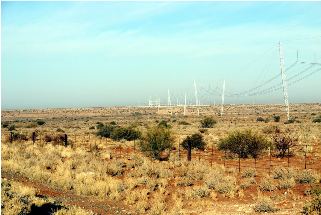
Plate 1, Existing Upington MTS and strategic high voltage power line viewed from the Lutzputs Road.
