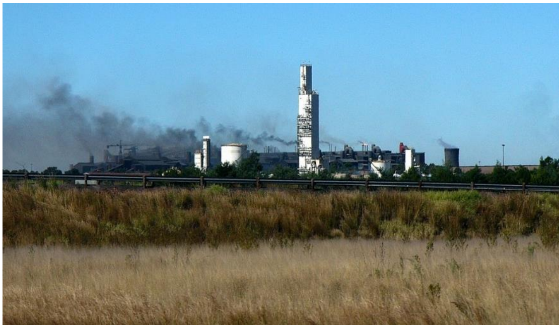
Figure 3: Evraz Highveld Steelworks located north-west of the proposed Transalloys PV Solar Facility
