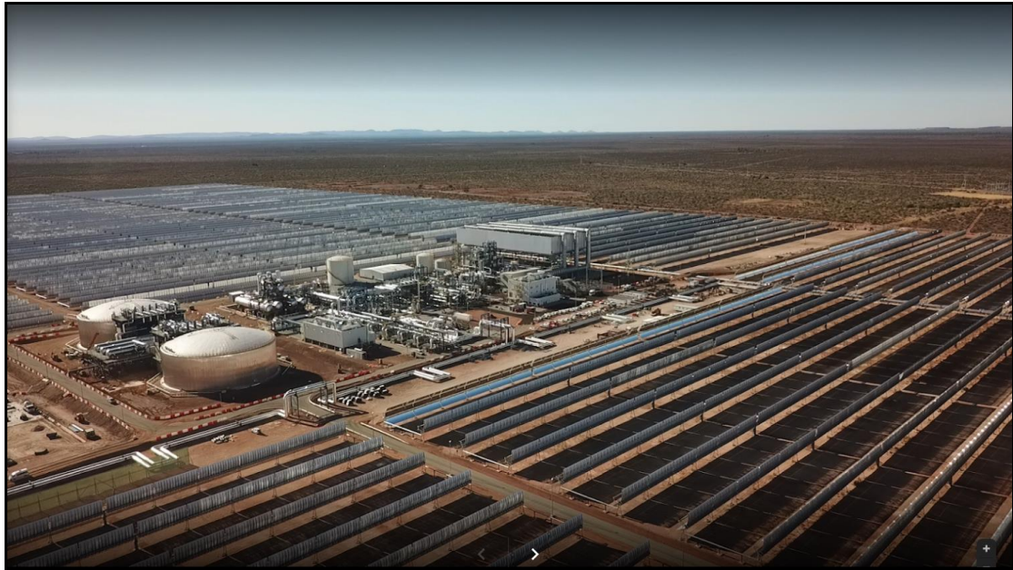
Figure 8: Kathu Solar Park (Photo: Google.com).
